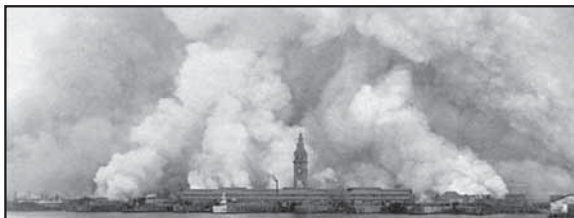
The fire that destroyed 500 city blocks after the 1906 quake raged out of control because liquefaction broke water pipes that were needed by firemen to fight the fire.
